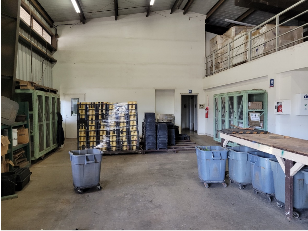
Figure 5: Western side of the existing Operations building
