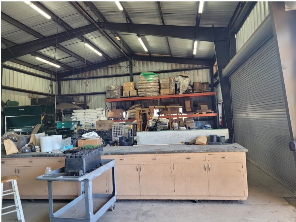
Figure 6: Eastern side of the existing Operations building
