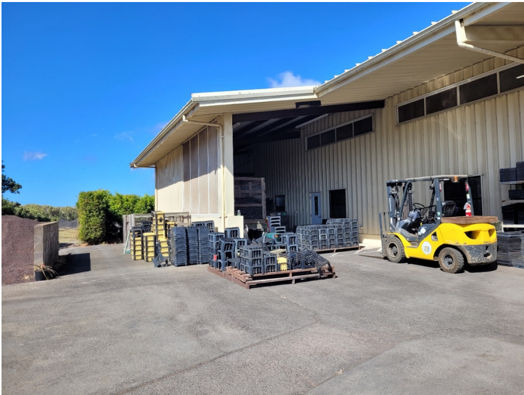
Figure 4: Covered exterior area of the existing Operations building
