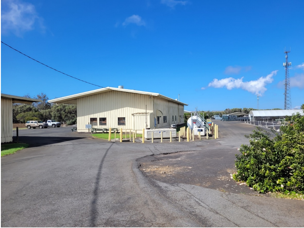
Figure 1: Paved entrance to existing Operations building
